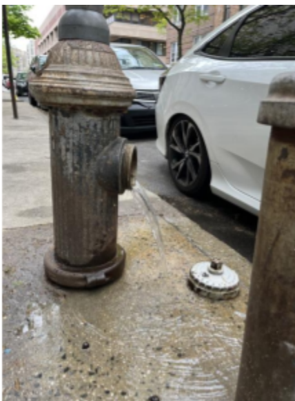
Figure 1: Open Fire Hydrant Losing Water Mata, Jenny (2023). Figure 1. April 29, 2023
